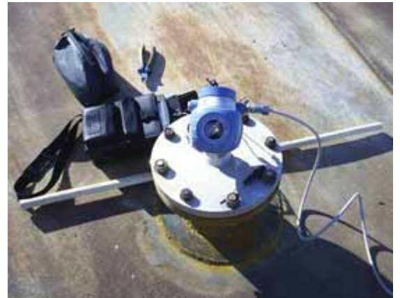
Figure 1: Rosemount 5401 installed on 7 m. (23 ft.) tall tank
